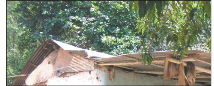
Pic. 17: Roof detail
