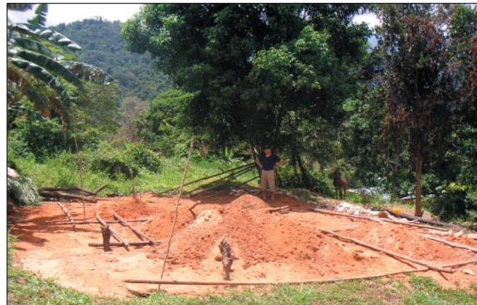
Pic. 15: A new construction site
