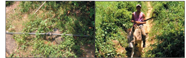
Pic. 3: fixed water pipe
