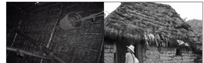
Pic. 20 Roof from inside
