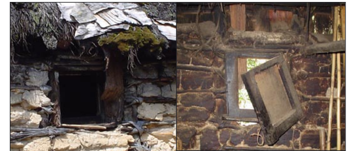
Pic. 18: Window from outside
