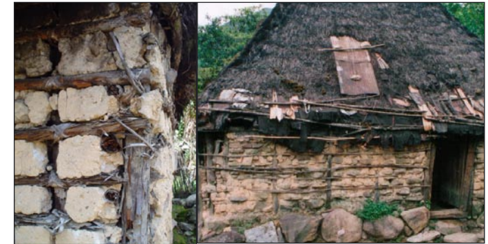
Pic. 16 Wall construction detail Pic. 17 Wall
