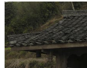
Pic. 16: roof covering
