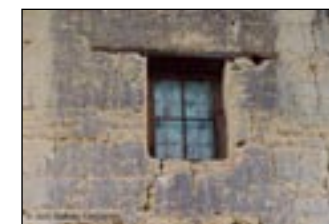
Pic. 4: outer wall of an earthrammed tulou, Zhenchenglou, Hongkeng
