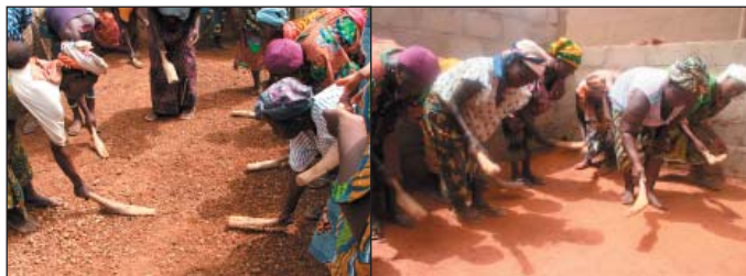
Pic. 13: Tamping of the loam floor
