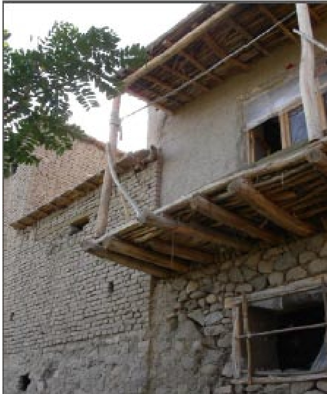
Pic. 12: Balcony construction
