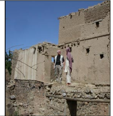
Pic. 15: Different walling types in one construction
