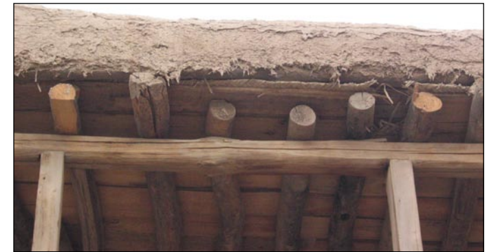
Pic. 16: Roof construction
